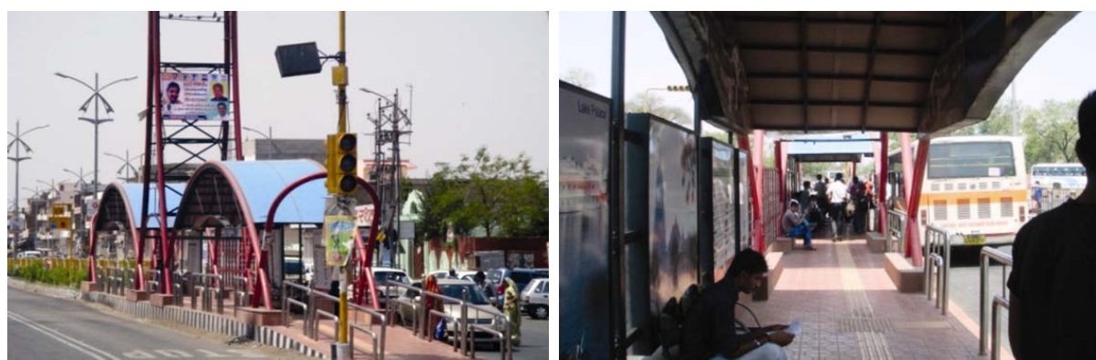
Figure 3.31 (Left) Design of the bus station with access ramp (Right) Station from inside
