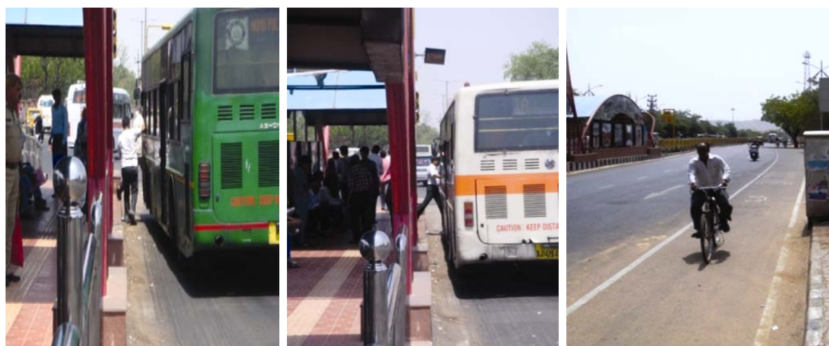
Figure 3.34 (1) Level-boarding problems (2) Bus distanced from the platform (3) Cycle track
