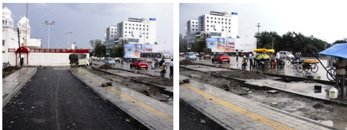
Figure 3.36 (Left) Footpath getting discontinued by a building obstruction (Right) Under construction
