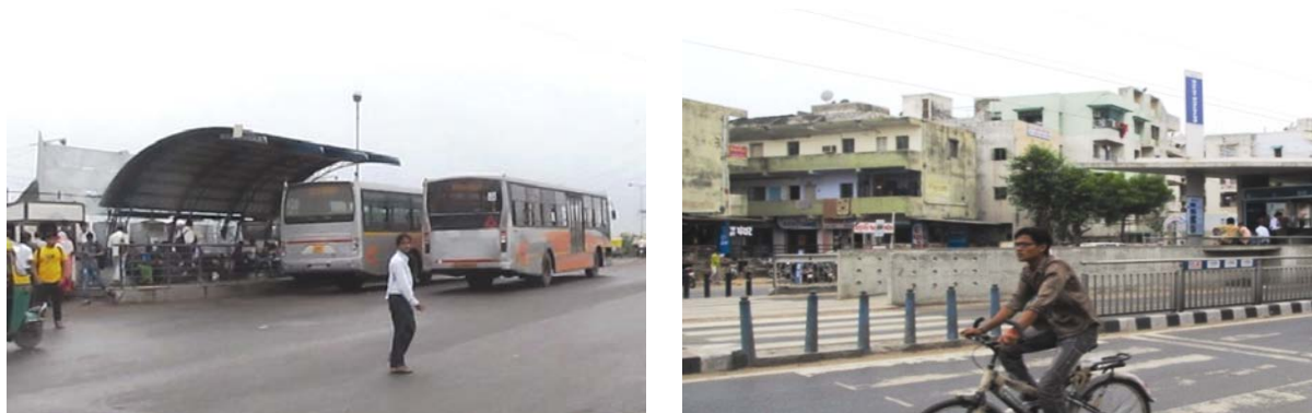
Figure 4.20 (Left) R.T.O. bus station: Low height, no ramp, no level boarding (Right) Concrete pillars at entry of station
