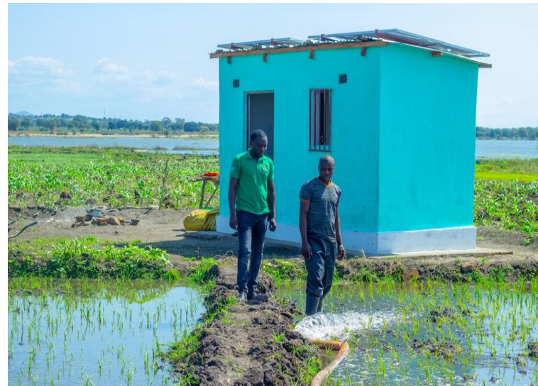
Kanyumba Irrigation package
