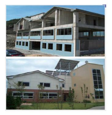
Figure 2.4 U-value 0.15 W/m2K Panel Approach system (PAS)
