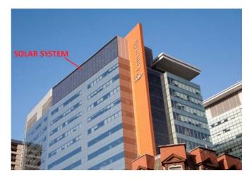
Figure 5.6 JMSB building façade with innovative solar façade system
